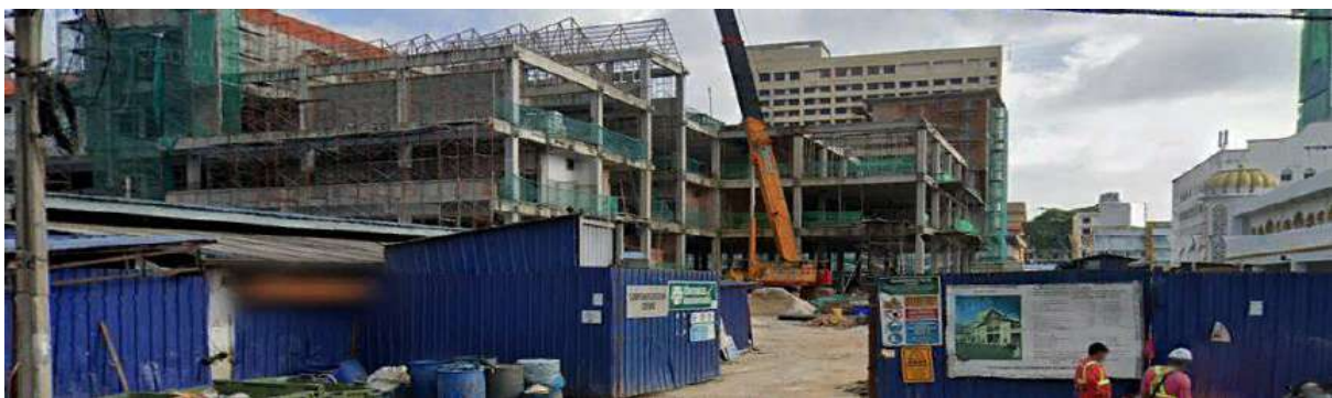
Figure 20: Ongoing project of 7-storeys Parking Block near the market
