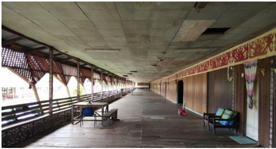
Public corridor space of the Longhouse. (picture taken during site visit in Kampung Kaban, 6th November 2018)
